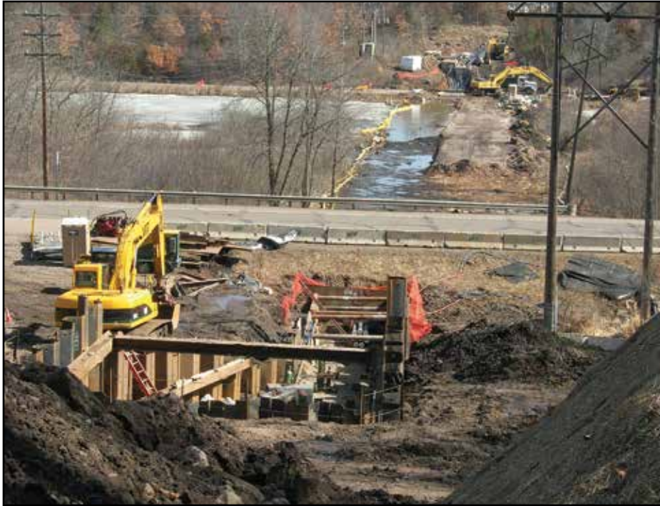
Don't forget to look at the big picture of the overall project when doing site inspections. Are the BMPs sufficient and working in concert to protect the total site?
